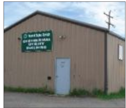
The Heat Exchange building should be celebrated.
