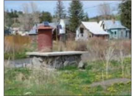
Water features exist throughout the Town of Pagosa Springs. The Bureau of Reclamation Gaging Station is shown above.
