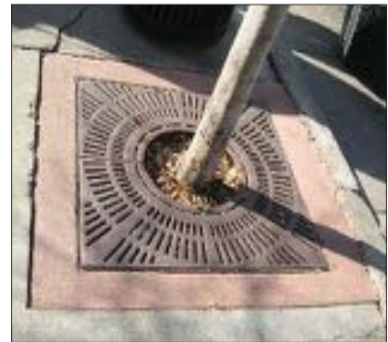
An existing tree grate in Downtown Pagosa Springs. A standardized tree grate should be selected to ensure uniformity along the public right-of-way and for efficient maintenance.
