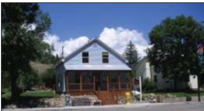
There are several residential structures flanking Highway 160 to the east of the Downtown Core that have been renovated to accommodate commercial uses.
