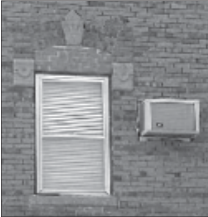
Do not locate window air conditioning units on a building's primary facade.
