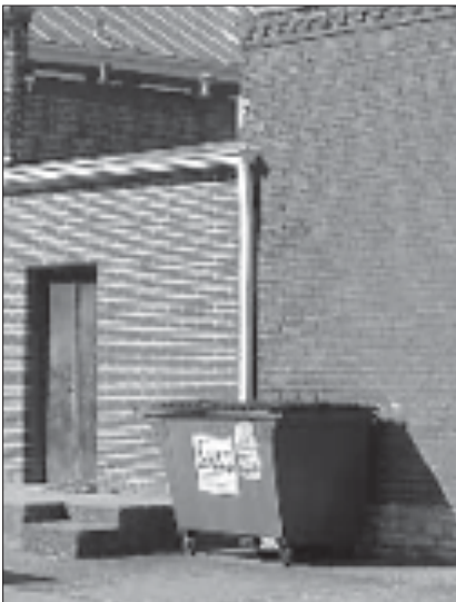
Where dumpsters are visible from a public way, they should be screened from view.
