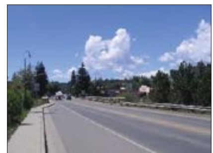
1st Street Bridge
