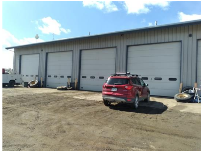
Figure 10: County Maintenance Facility
