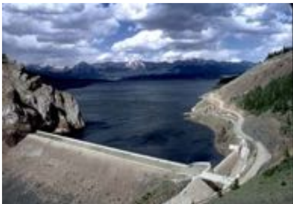
Taylor Park Dam and Reservoir - USBR photo
