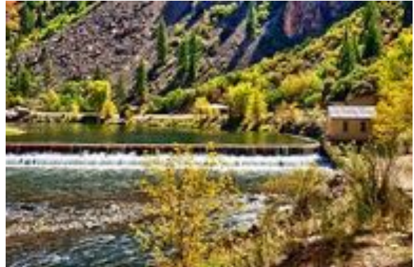
East Portal of the Gunnison Tunnel
