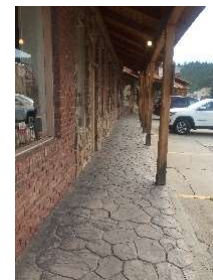
The sidewalk in front of the stores is stamped concrete
