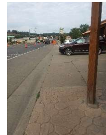
Consider landscaping to direct pedestrians onto the sidewalk to the right
