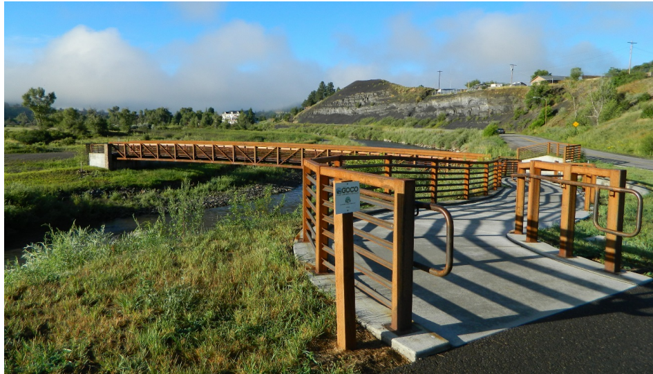
Pedestrian Bridge at 6th Street
