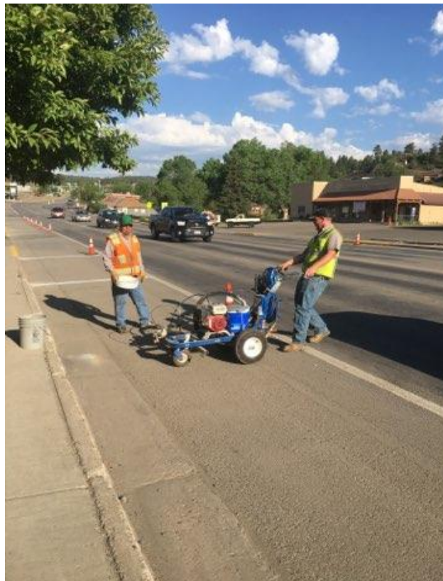
Streets Employees Frank Mestas and Blair Crook Paint New Parking Stall Lines
