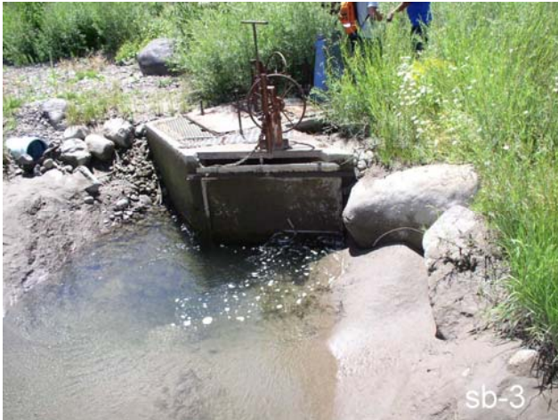
Older intake structure at West Fork of the San Juan River
