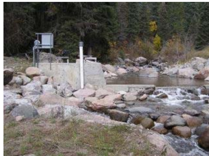
Diversion and intake from Four Mile Creek
